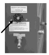
Open water flow valve 1 ¼ turns to allow water to fill reservoir.
