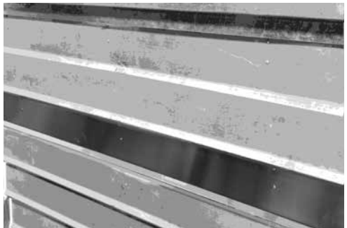
Fig.9 - New louver vane installed
