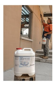
\*NOTE: Once Stabilised Earth Water Repellent is applied, it creates a waterproof seal and will not allow other sealers to penetrate the surface. Do not apply to internal walls or the final application of Earth Binder will not penetrate and will leave an undesirable milky appearance.
