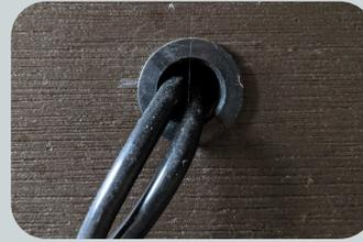
Plug and play models have designated electrical panels so please keep this in mind when placing your tub in its location. All 240V hot tubs allow you to choose which panel you would like to drill a hole into for your wiring to pass through.
