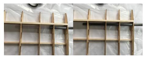
35. Trim the wing tip balsa sticks and splice 2MM balsa sheets
