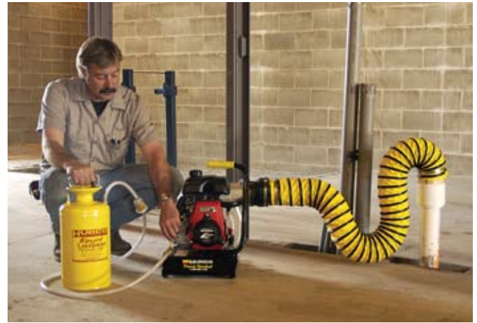
Typical set up for Smoke Testing
