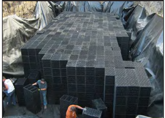
INSTALLING FLO-CELL® CAPPING LAYING OVER TANK MODULES
