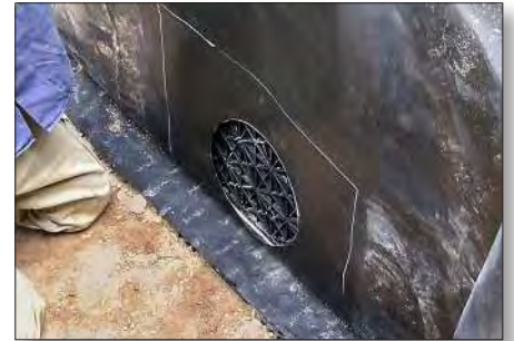
3. Cut the opening for the pipe
