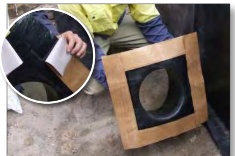
6. Peel the back corner of the flange to expose the sticky side
