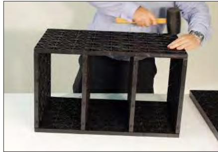
Use a rubber mallet to hammer the pins to ensure a tight fit.
