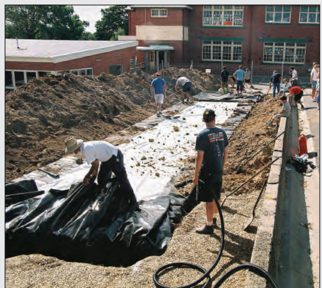
Liner is pulled up over the constructed tank.
