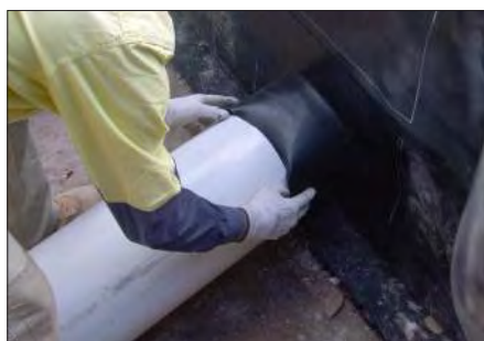
8. Insert the pipe and push all the way against the tank
