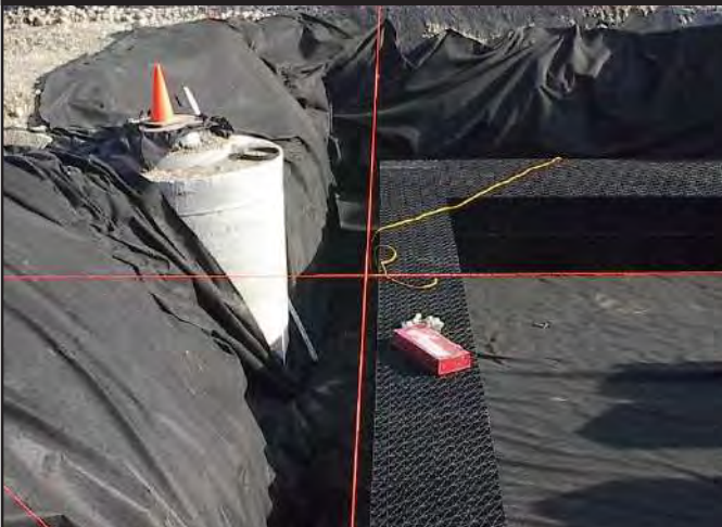
STRING LINES FACILITATE INSTALLATION OF BASE LAYER
