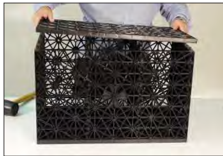
Flip the module over again and repeat the last step.
