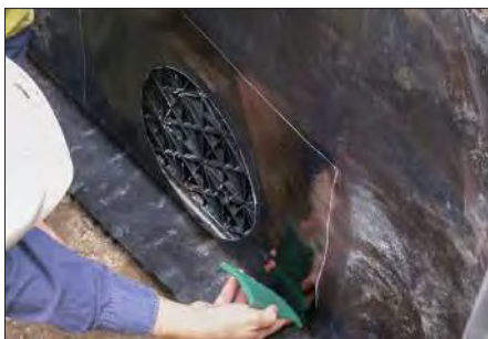
4. Prepare the area of the boot flange with a polypropylene glue
