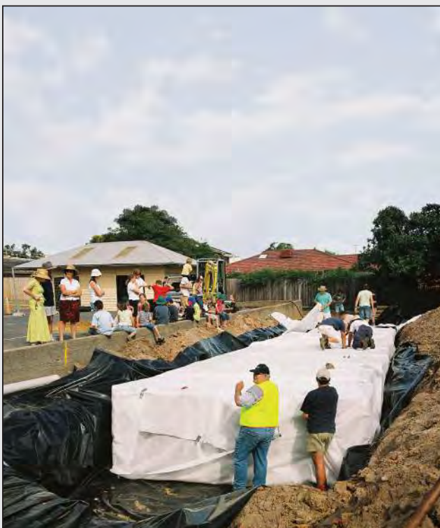
Constructed tank is wrapped in geotextile.
