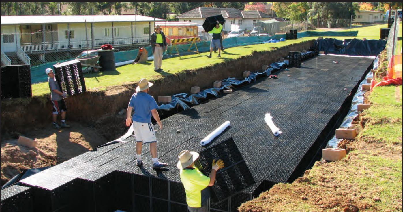
INSTALLING TANK MODULES
