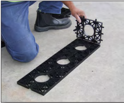
Clip first divider into long plate. Ensure the irrigation channel on the long plate is facing the ground.
