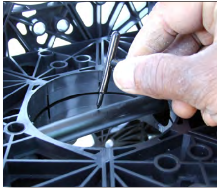
Puncture the poly irrigation pipe from the top first
