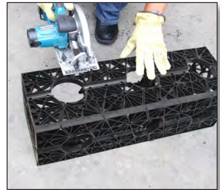
Cutting the module with a circular saw
