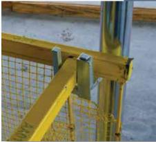
Tie Down's Edge Fall Protection System (EFPS) is a safe and efficient way to protect workers from leading edge fall hazards. EFPS is wind tunnel verified up to 110 mph and meets both OSHA and ANSI requirements.
