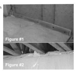
details. Trim any excess insulation for a neat appearance. Pull the release paper from the factory applied double stick tape. Overlap this 6" facing tab and adhere to the adjacent blanket. **Option #2**
