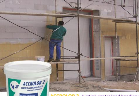
ACCROLOR 2 - Suction control and bonding agent for the regulation of high and low suction substrates. For external and internal use.
