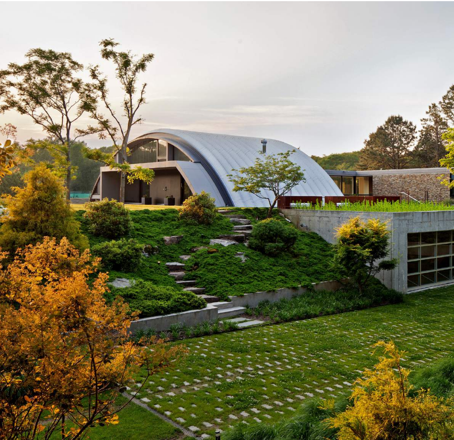
ARC HOUSE, USA ARCHITECTS: MAZIAR BEHROOZ OCHRE ROCK PANELS
