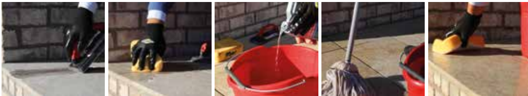
PIC 1. Fill joint with grout.
