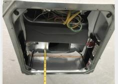
Measure the plenum depth. With Mounting Bracket attached . 5 1/8 Plus or minus 1/8 Without mounting bracket attached– 5 7/8 Plus or minus 1/8
