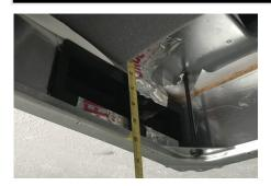
Vertical location of the ductwork (From bottom of AC to top of ducting) With Mounting Bracket attached 2 5/8 Plus or minus 1/8 Without Mounting Bracket attached 2 7/8 Plus or minus 1/8
