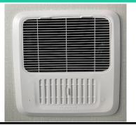
Remove air conditioning ceiling assembly. Remove all components unit you have full access to the plenum area.
