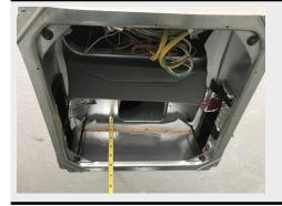
Measure the plenum depth. With Mounting Bracket attached . 5 3/8 Plus or minus 1/8 Without mounting bracket attached – 5 5/8 Plus or minus 1/8
