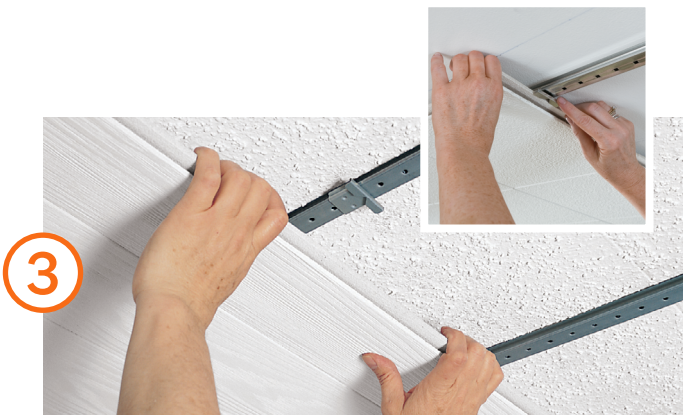
3 Position tiles or planks; slide and secure clips
