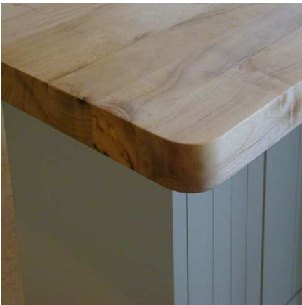
Myrtle Plank Installed
