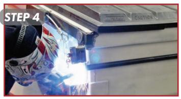
On the left arm, turn the key to the right, releasing the chain. This will allow you to open the **LIDOLOK**, Using the front of the container as your level, cut the 1" O.D. pipe the exact length you need, and tack the pipe to the left arm as shown above. Make sure that the arms are vertical, allowing the pipe to move up and down freely.
