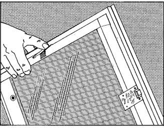
5. Attach new clips to new sash. Use flat clip on top rail. Self-spacing clips are used on sides and bottom rails.
