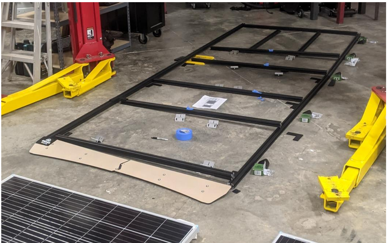
Figure 2: Layout rack on floor including hardware, label parts, hardware quantity, and locations as needed. *Note image above is from a different rack kit
