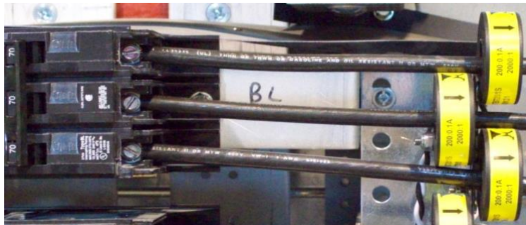
Typical i-meter®636 Installation
