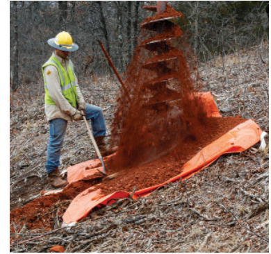
RDB-8x8-22V in Action Installing a Utility Pole
