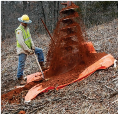
RDB-8x8-22V in Action Installing a Utility Pole
