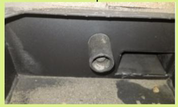
Locate the set screw that holds the igniter rod clamps in place. These are accessible through the removable side panels
