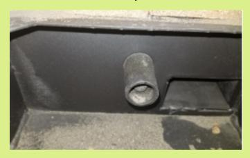
A proper positioned igniter rod will be as directly centered as possible inside the tube, and be inset back from the opening about %"
