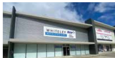
WA Store & Warehouse
