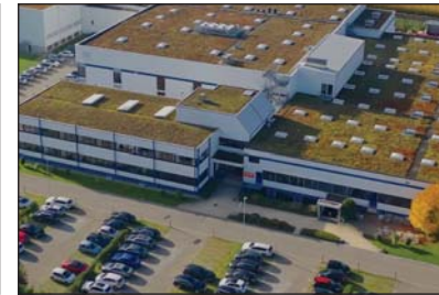
IQAir AG Technology Center Steinach, Switzerland
