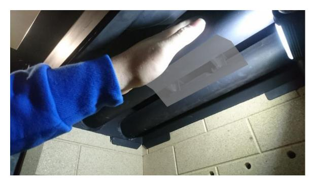
Once the flue has been swept, please remember to slide the throat plate back into the center of the heat exchangers.
