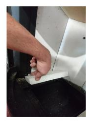
Remove grate and base fire bricks.
