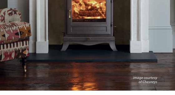
Another function of the superimposed hearth is to provide a physical/visible barrier marking the clear areas required around the appliance. This is often achieved with a change in surface height or texture and serves to warn against fixing any combustible flooring such as carpet, wood or laminate within this protected zone as well as the casual placing of anything combustible. This also helps to warn occupants they are near a hot appliance and mitigates possible burning.
