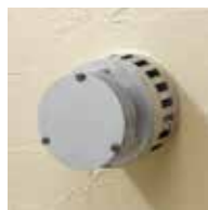
Balanced Flue (No chimney required) BF
