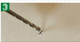
Using your drill with the 3/8" bit; drill the hole for your rubber tee starting from the back of the turf.
