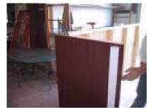
Install panel E. Keep the top walls level and push in the bottom.
