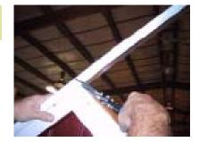
Install the dripedge, which can be purchased at your home improvement store. You can then use tin snips or sidecuts to cut the dripedge so it fits over the angles of the roof. Fasten with 3/4" roofing nails.
