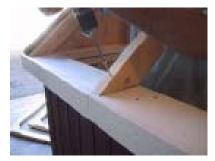
Install trusses in premarked spot. Note: trusses only come to the edge of the 2x6. You may have to pull them to the correct position. This is from not fastening the gussets correctly or from bowing wall or other factors.
