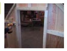
Install (3) 2'x3'x36" pieces over top of the door and sides of joints. This will provide strength for the door. Keep even with the edge of the door.
