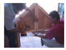
Next fasten panels G and H together. Note: keep the edge even. This will be the top of the door so this is very important. The trim should got to teh bottom as can be seen in the picture. 18
