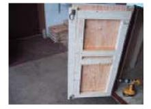
Install left door using spacer bar to provide the correct spacing. And install door stops as shown.
