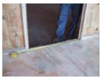
When installing panel F measure the distance between the 2x3's. Make sure this measurement is 34". If it is NOT 34", adjust the panels until it is. Otherwise, there will be problems when installing the adult door.
