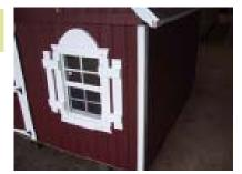
Install the corner trim using small white nails. Be careful to not "wrinkle" the corners when installing. Tip: do one side while pressing in, than do the other side. 78
