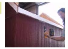
Fasten small blocks on bottom of 2x6. This will provide strength.
