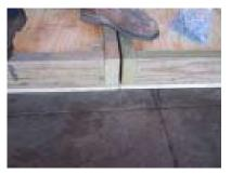
Make sure the plywood is even before fastening! If it is not you will have an uneven floor, and it could cause problems later.
