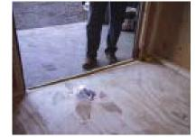
Measure between the door fom 2x3 to 2x3. The measurement should be 40". If it is different adjust until it is. You may have to loosen the outside walls and move the slightly. (variation in wood widths)
