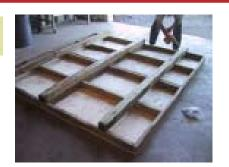
This shows the optional 4x4 runners, you will need to have 3 in order to have 1 under the center joint. if you use 2 the floor will sag. Note: These are optional, but it will aid in moving the building later. If you are adding a Deck & Rail you MUST add these! Other wise the small door will not clear the deck.
