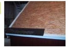
Read your shingle pack for installation instructions. You can use a utility knife to cut these both with a striaght blade and a hook blade. Cut tabs off of the shingles and install a starter strip. Notice the glue strips toward the bottom. Fasten with 3/4" roofing nails.
