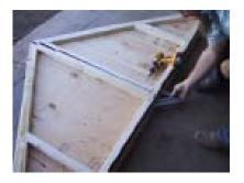
Fasten panels L and M to each other. Make sure they are even on the bottom. Piece may bow slightly
