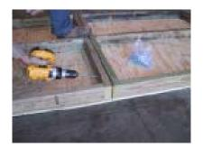
Screw the sections together. Put two screws in from each side for a total of 4 screws, one towards the plywood and one towards the top. Repeat this roughly every 8" to 10" apart. 2
