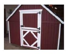
Install the top of the door, centering it between the top door trim and the bottom half of the door. Install latch. 80
