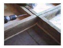
Continue to make sure the plywood is even at the bottom. The 2x4 may vary in width at times.
