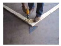
Fasten truss gussets, keep top even. Install one gusset on either side of the truss. Make sure the gusset does not stick out past the truss, or roofing will not fit.
