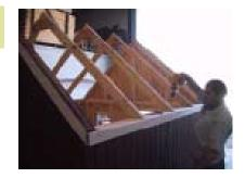
This shows an 8x8. An 8x10 and 8x12 will have extra trusses. The trusses are positioned every 2' on center (or to the middle).
