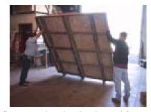
Turn the floor around so that the plywood faces up. Make certain that the ground is level where the floor sets or you may have problems with panels or roof. You will need several to do this, do this with caution. Do not stand under the floor.
