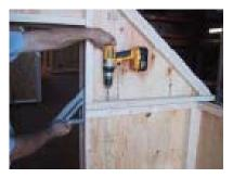
Keep the edge of the door frame even and push in the trim against the siding. Fasten.
