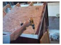
Install the first sheet of OSB sheeting. It will start at the edge of the endwall truss. There will be a 1/2" gap between OSB and 2x2.
