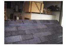
Install the ridge cap on the top as shown. Use 7/8" roofing nails to fasten these.
