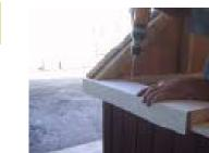
Install the other side of 2x6 with trim. In the case of an 8x10 and 8x12 there will be an additional piece to install.
