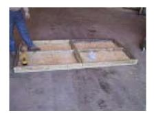
Thank You For purchasing from Little Cottage Co. Please note: the following pictures are from the construction of an 8x8, 8x10 and 8x12 units may vary slightly. Lay (2) 4x4 flooring sections side by side. Make sure it it on a level area.
