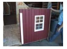
Next Install panel I. Keep the top wall level and push in at the bottom.
