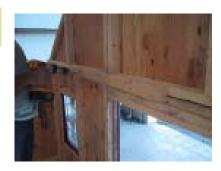
Install the  $2^{\circ}x3^{\circ}36^{\circ}$  brace over joints. If you are installing a loft you will have to take this off. The loft will then provide support.
