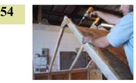
Fasten onto the truss. Remember it will only come to the center of the truss. This will allow room for the next sheet of OSB. You may have to move the truss from side to side
