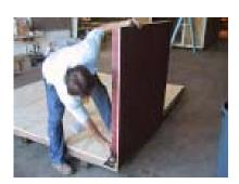
Install section A. Then install section B. And in the case of an 8x10, 8x12 install section 2B. Repeat on the other side. And again if it is a larger size you will have section 2C to assemble. 8
