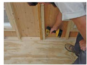
With the section in place, drive a 2½" screw through the 2X and into the floor section.
