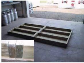
Locate a level spot and lay the two (2) 4'x4' flooring sections side by side. Verify that the plywood sheets are level to ensure that floor is even.
