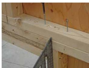
At the lower section's upright 2X, verify that the upper and lower sections are flush. Drive two (2) 2½" screws through the upper section's base 2X and into the lower section. Repeat above the opposite upright.
