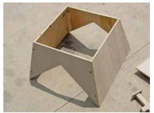
Now assemble the two sections together, noting that abutting edges must be caulked as shown in preceding steps.
