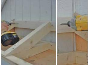
Secure the awning to the structure using four (4) 2½" screws along both the top 2X and the bottom 2X.
