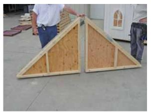
Locate the upper rear section panels as shown above.
