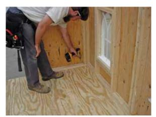
Using a square to ensure the top of abutting sections are flush, drive a  $2\frac{1}{2}$ " screw through the bottom 2X and into the floor section.
