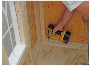
Set a level atop the abutting corner and ensure joint is flush. Drive a 2½" screw through the base 2X and into the floor section at the corner of back panel section
