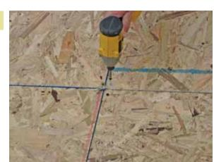
Place the next OSB sheet in place and secure the lower left corner with a 11/4" black head screw.
