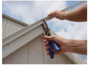
Continue to attach dripedge to the peak. Then, snip the dripedge to accommodate the bend.
