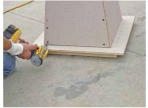
Secure the steeple to deck with two (2) 11/4" screws on all four sides.
