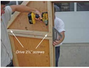
With the upper section in place, verify that the upper and lower inside 2X's are flush. Then drive 2½" screws through the upper section's base 2X and into the 2X below as shown.
