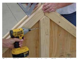
Drive a 2½" screw through abutting 2X's near the top.
