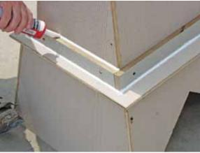
Run a bead of caulk along the upper and lower perimeters of the trim as shown.
