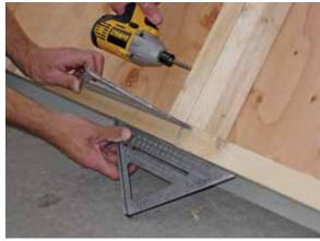
Using a square to ensure that sections are flush, drive a 2½" screw through the abutting 2X's several inches from the bottom.
