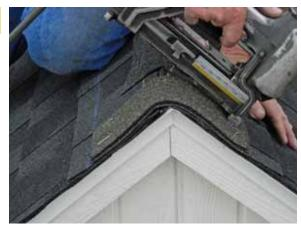
Then, align with both the chalk line and end of structure and attach to roof.
