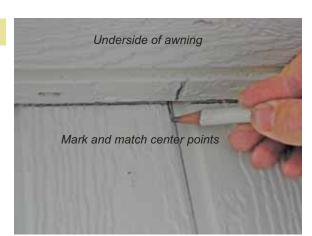
Measure and mark the center point on the underside of awning. Holding the awning, match the center points and align the bottom of awning with the line. If desired, lightly trace the awning for clarity.
