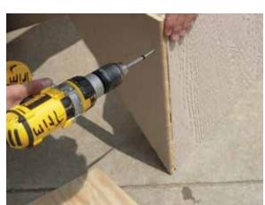
Again position the two pieces together and secure using two (2) 11/4" screws.
