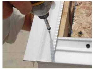
Locate the residual dripedge previously trimmed and attach as shown above.
