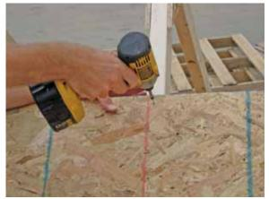
Once on center, drive a 1½" black head screw through the OSB and into the center line of truss.
