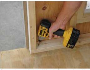
Secure the panel's base 2X to the floor section with a 2½" screw. Likewise, drive screws along base 2X every 16", as applicable.
