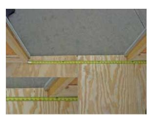
Set the corresponding back well section in place. Verify that the opening between the inside 2X's is 34". If not, adjust front panel section slightly while making sure that it does not overhang the corner of floor section.
