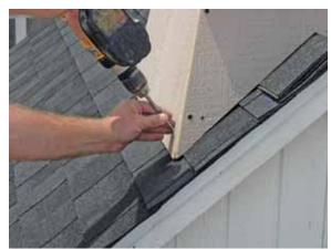
With assistance, carefully lift the fully assembled steeple to position and secure by toenailing a 2½" screw through the steeple and into the roof at each corner.
