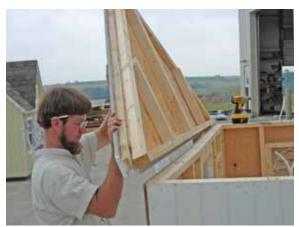
Carefully set the upper rear section in place, with the base 2X set squarely atop rear panels.
