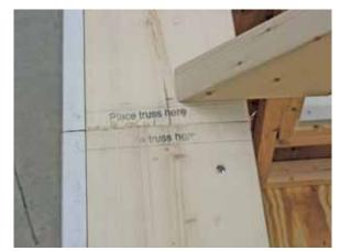
Beginning at one end of structure, raise the first truss into position. Note that all truss locations are marked on the eave plates.
