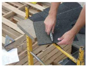
Prepare to cap the roof by trimming the first cap section to the proper width.
