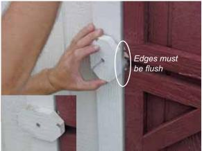
Locate the wooden door latch and position lengthwise as to allow its edge to be flush with the door trim. Drive a 2½" screw to the point at which the latch is tight - but loose enough to turn by hand (see Inset).
