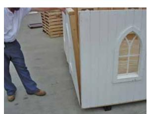
Locate the corresponding front panel section and set in place.
