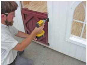
Set lower section of door in doorway and atop the door bar spacer. Make sure the narrow gap on both sides of door is equal. Then secure using 11/4" black headed screws as provided in your package.
