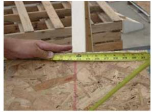
Verify the next truss is 24" on center, slightly adjusting left or right as needed.
