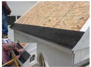
Attach the first row of shingles, trimming off excess as shown in the inset.
