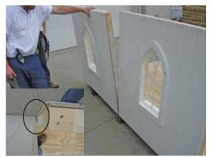
Locate the next panel and set in place. Note that the lip on the next panel should overlap the section previously secured.
