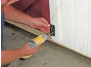
Set the lower section of rear door in doorway, allowing a narrow gap between the door and floor. Make sure the narrow gap on both sides of door is equal and secure the lower hinge using black headed screws.
