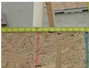
Again measure 24" on center from the previous truss, and adjust slightly as needed.
