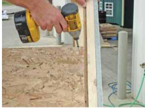
Secure the <u>upper and lower (right) corners</u> of the OSB.
