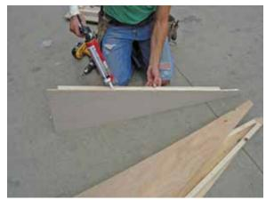
As with the base, assemble the steeple portion by first caulking along the edge of one side.
