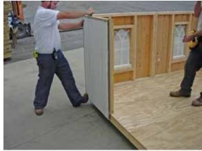
Now locate a rear panel section, set in place and apply pressure to the bottom.
