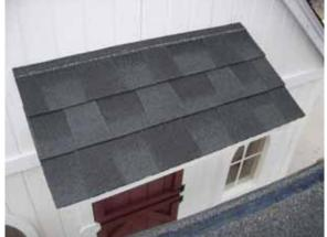
Attach the final shingle, trimming off excess along the awning. The awning is now complete.
