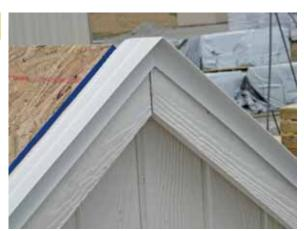
Bend as shown above and secure dripedge along the downward edge using 11/4" screws every 2'. However, DO NOT secure the last 12" of dripedge.
