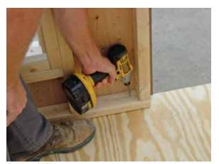
Drive a 2½" screw through the base 2X and into the floor section along the door opening. Screws should also be driven every 16".
