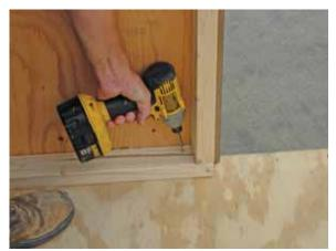
Drive a 2½" screw through the base 2X and into the floor section along the door opening. Screws should also be driven every 16" along the base 2X.
