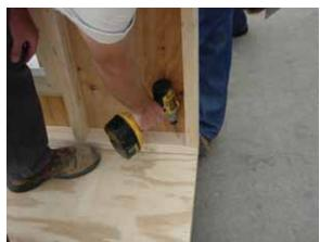
Next, secure the outer edge of the panel to the corner using a 2½" screw. Then, drive additional 2½" screws along the base 2X every 16."
