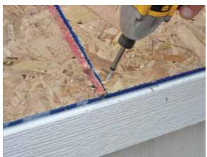
Place the next OSB in place, align edges, and secure the <u>lower left corner</u> to the underlying truss using 1¼" black head screws.
