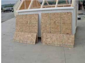
Locate the Orient Strand Board (OSB) and place in a convenient location. Note the actual number of OSB panels will vary based on the length of your structure. Refer to your layout diagram.
