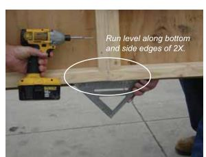
Using a square to ensure that sections are flush (both as shown and along the edge of 2X), drive a 2½" screw through the abutting 2X's several inches from the bottom.
