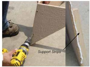
Position the two pieces as shown and secure using two (2) 11/4" screws. Note that screws must be driven into the 1X support strips as shown.
