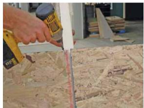
Proceed to the next truss, which will hold the OSB splice. Again, slightly adjust to allow the edge of OSB to be centered on the truss and drive a 1½" black head screw.
