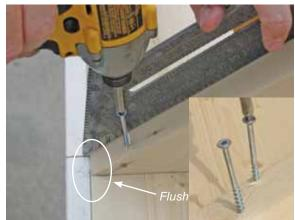
Using a square, verify that the end of truss is flush with the edge of eave plate. Secure using two (2) 2½" screws.
