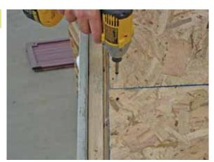
Place the upper row of OSB in place, align, and secure the <u>lower left corner</u> with a 1½" black head screw.
