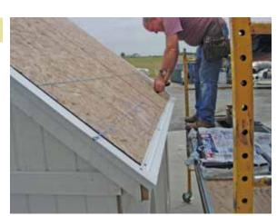
To prepare to shingle the roof, first measure upward from the edge of dripedge 8¼" and snap a chalk line.
