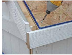
Once properly aligned, secure the <u>lower left corner</u> of OSB to the underlying truss using a 1½" black head screw.
