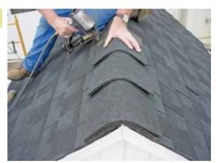
Continue capping roof until reaching the opposite end of structure. However, do not attach the last cap section.
