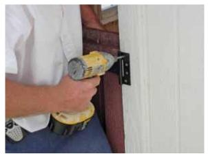
Attach upper hinge of rear door as shown. Then, verify that door opens and closes freely.
