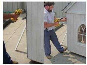
Similarly, secure siding at abutting corners using 1½" screws every 8". Then attach the corner trim as shown.
