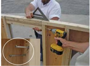
Level the block using a square and secure using two (2) 2½" screws on both ends.
