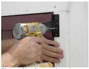
Attach upper hinge of upper rear door as shown. Then, verify that door opens and closes freely.
