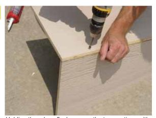
Holding the edges flush, secure the two sections with  $1\frac{1}{4}$ " screws every six inches.
