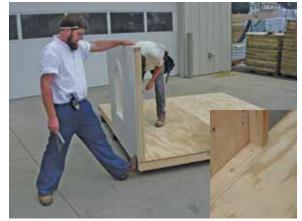
Repeat on the opposite end of panel. Then, secure the panel using 2½" screws every 16" between.
