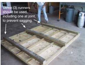
4' x 4' runners (as shown) are <u>optional</u> on standard unts. However, runners are necessary when adding a deck and rail to ensure child door clears the deck.
