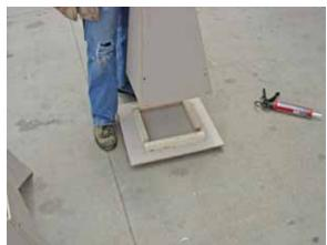
Set the completed upper section of steeple on the steeple deck as shown above.
