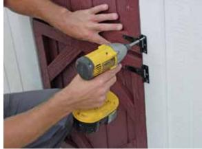
Next, set the top door section in place atop the lower door section. Note that you should leave a ¼" gap to allow doors to open and close independently. Then, secure door using 1½" black headed screws.
