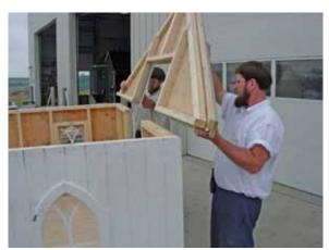
Carefully set the upper front section in place, with the base 2X set squarely atop front panels.
