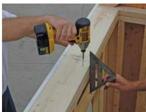
Attach the next trim section, ensuring that it is flush with the inside of the side wall's 2X.
