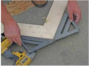
Use angles to square the joint of the truss, making sure the tips are even.
