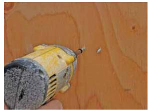
From the inside of structure, drive corresponding 1¼" screws through the side wall and into the 2X's on awning.
