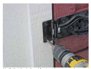
Verify that the bolt and front catch are properly aligned. Then, tighten the front catch.
