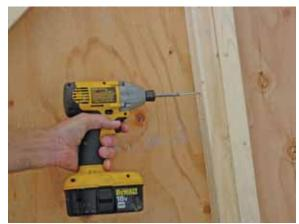
Drive a 2½" screw near the mid-point of abutting 2X's.
