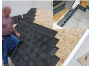
Continue to stagger shingles, working up to the ridge and towards the opposite end of the structure. Once at the ridge, carefully trim excess shingles to expose ridge opening (see inset). Repeat on opposite side.
