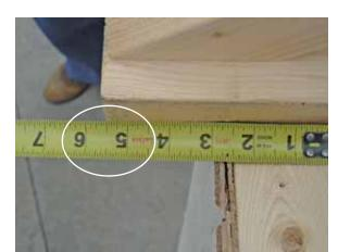
Note that both ends of the upper section must overhang the innermost edges of the side wall 2X's by 5½."
