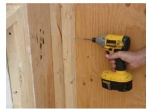
Drive a 2½" screw through the mid-point of the end 2X (and into the abutting 2X).
