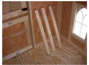
Locate the three (3) 36" door braces provided in your package. These 2X supports brace the joint between the upper and lower rear wall sections.
