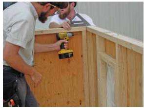
Keep the level on top of the side and rear panel sections and drive a 2½" screw through the end 2X and into the abutting 2X.
