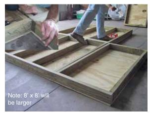
As applicable, set additional sections in place and ensure that abutting plywood is level. Then, secure sections as previously described.
