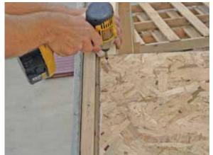
With the lower row of OSB in place, proceed to the next row. Align the OSB as with the preceding row and secure first the <u>lower left corner</u> followed by the <u>upper left corner</u>.
