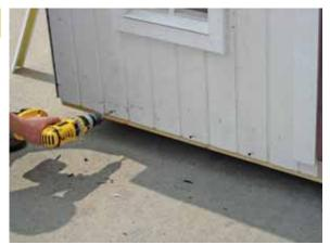
Secure the bottom of siding to the floor section using  $1\frac{1}{4}$ " screws every 8".
