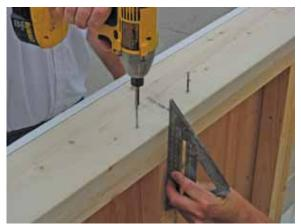
Note that screws should be driven on both sides of wall splice as well as every 16".
