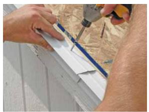
The residual dripedge should be slid below the ascending dripedge and secured with a 1½" screw. Repeat attaching dripedge on the opposite end of structure and on the awning.
