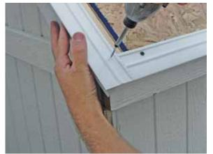
Hold the next strip of dripedge along the end of roof line and secure as shown above.
