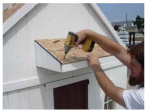
Attach OSB to the awning, securing with 11/4" screws at all corners and every 6".
