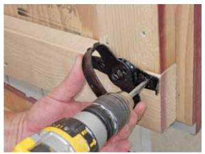
Secure the pin handle using the 11/4" black headed screws provided in the package.
