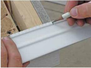
One piece of dripedge will need to cut to the proper length. Do not discard the residual dripedge, however, as it will be used on the opposite side of the structure's roof.
