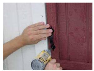
Attach the upper and lower outside pull handles using black headed screws.
