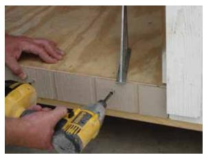
Locate the strip of siding to be attached below the rear doorway. Set in place, using an angle to ensure that the top of strip is even with the floor of structure, and attach using four (4) 1½" screws.
