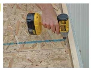
Repeat for the <u>lower left corner</u>. Then, drive 1¼" black head screws every 6" around the perimeter of all OSB sheets. Once complete, repeat for the opposite side of structure.
