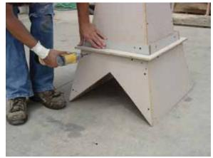
Secure the steeple to the base using two (2) 11/4" screws on all four sides.
