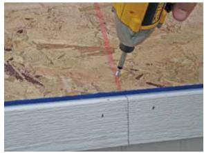
Now secure the center of the OSB to the underlying truss in a similar manner.
