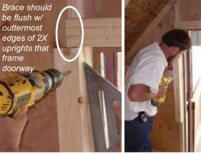
Use a square to ensure that the supports are aligned with the underlying 2X's. Attach one support above the door (from 2X to 2X) and the other two along the sides
