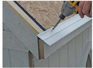
Set the dripedge along the base of roof as shown above, securing with 11/4" screws every 2'.
