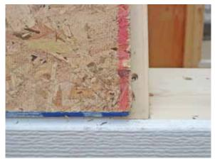
The lower right corner will reach, but not surpass, the center of the truss.
