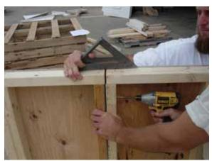
Using a square to ensure the sections are flush, secure the top of the abutting 2X's using a 2½" screw.
