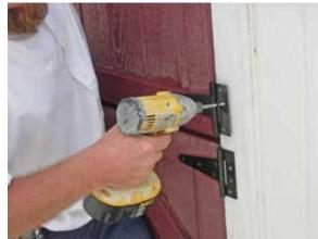
Set the upper section of rear door in doorway, allowing a narrow gap between the doors. Make sure the narrow gap on both sides of door is equal and secure the lower hinge using black headed screws.
