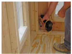
Drive a 2½" screw through the base 2X and into the floor section at the corner of panel.
