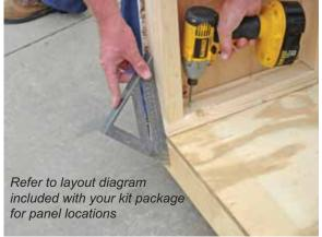
Set first side panel in place, using a square to ensure that it flush with the edge of floor. While applying pressure from the outside, drive a 2½" screw through the 2X and into the floor section.
