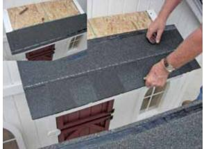
With the main structure now shingled, proceed to the awning. Attach the first (see inset) and second shingles.
