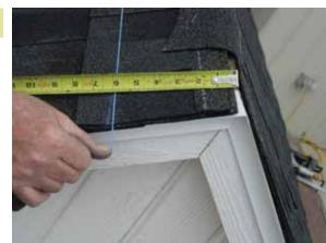
Measure downward 6" and snap a chalk line along one side of the roof.
