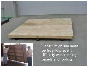
Once complete, turn floor on onto runners. Again, make sure spot is level or you may have difficulty when setting panels and roofing later.
