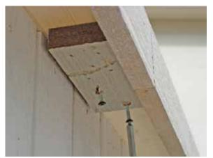
Attach the eave joint blocks (to the eave plates) on the underside of each joint using 2½" screws on both sides of splice.
