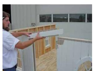
Locate the header block and set in place as shown.
