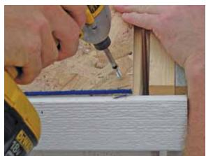
As in the preceding step, secure the <u>lower right corner</u> of OSB
