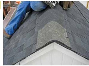
Instead, finish the cap using a no adhesion strip as shown.
