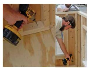
Using a square to ensure the top of abutting sections are flush, drive a  $2\frac{1}{2}$ " screw through the bottom 2X and into the floor section.
