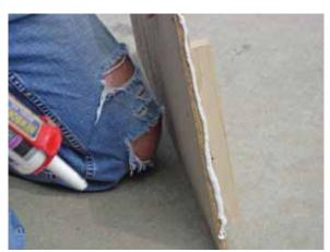
Beginning with a section without the ridge cutout, caulk the end as shown.
