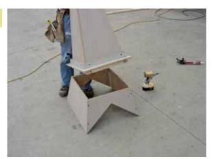
Set assembled steeple and deck on top of the steeple base as shown.
