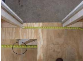
Set the corresponding front wall section in place. Verify that the opening between the inside 2X's is 20". If not, adjust front panel section slightly while making sure that it does not overhang the corner of floor section.
