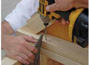
At one side, verify that upper and lower section's 2X's are flush using an angle and secure with a 2½" screw.
