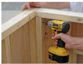
At the top, drive a 2½" screw through the section's end 2X and into the abutting 2X.
