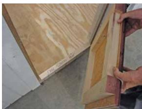
Locate the door bar spacer and insert along the floor between the door jambs.
