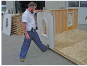
Locate a front panel section, set in place and apply pressure to the bottom.
