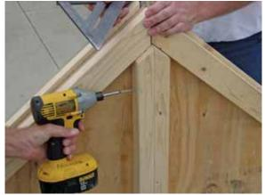
Drive a 2½" screw through abutting 2X's near the top.
