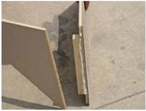
With the remaining section without the ridge cutout, caulk the edge as shown.
