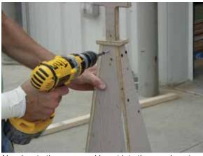
Now locate the cross and insert into the opening at the top of the steeple. Drive a 1¼" screw through the side of steeple and into the underside of cross, securing it in place.
