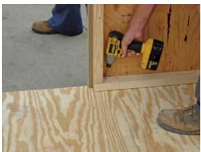
Drive a 2½" screw through the base 2X (at the doorway) and into the floor section. Likewise, drive screws along base 2X every 16", as applicable.
