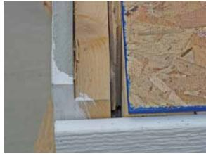
Beginning at the <u>lower left corner</u>, align the first OSB sheet with the edge of truss. Likewise, use an angle to ensure that the bottom edge of OSB does not exceed the tip of the truss.
