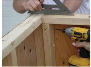
At the top, then drive a 2½" screw through the section's end 2X and into the abutting 2X.
