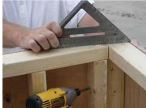
With the square held in place, drive a 2½" screw through the corner 2X and into the abutting section's 2X.
