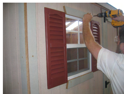
Install the trim above and below the shutters.
