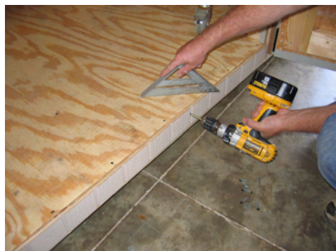
Install the siding strip beneath the door. Be sure to keep even with the floor as shown with the square.
