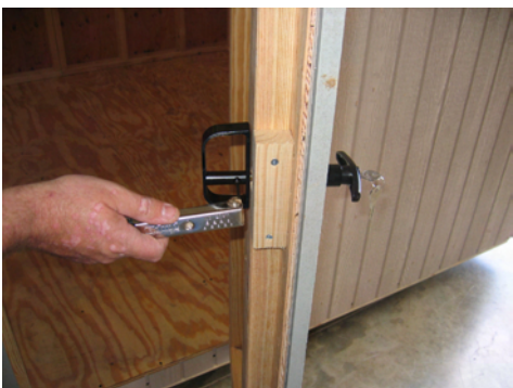
Install part D of the door latch on the inside.
