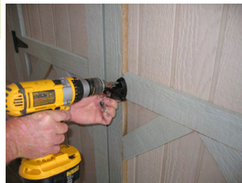
Install the door latch in predrilled hole.
