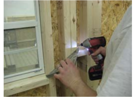
Secure wall splices with 2 1/2" screws.
