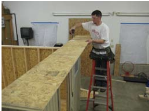
Secure front wall overhang with 1 1/4" zinc screws every 6 to 8".
