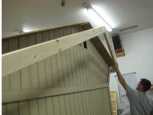
Install rake as shown
