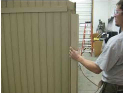
Next install trim on back corners.
