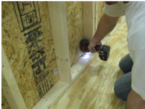
Secure back wall with 2 1/2" screws.
