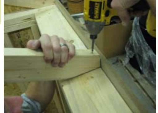
Once truss is in place secure with 2 1/2" screw.
