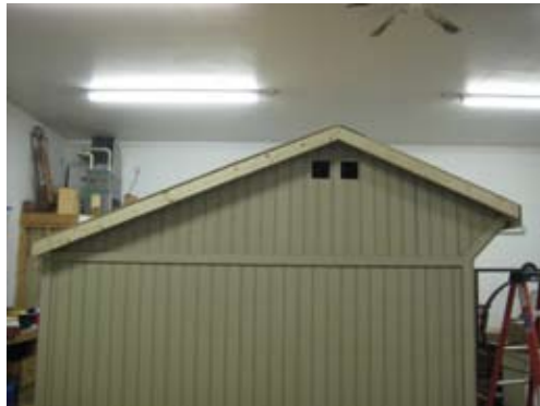
Rake is completed.
