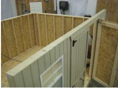
End walls complete.
