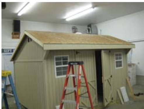
Sheathing is completed and ready for shingles.
