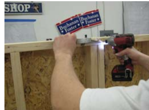
Secure top end with 2 1/2" screws as shown.
