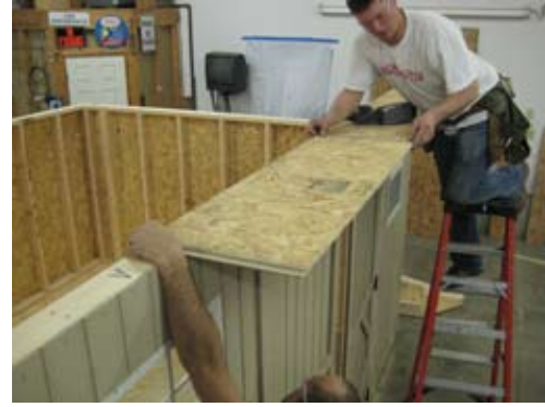
Continue with front wall overhang.
