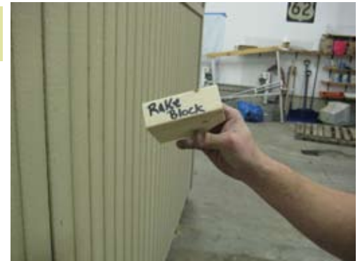
Locate rake block.
