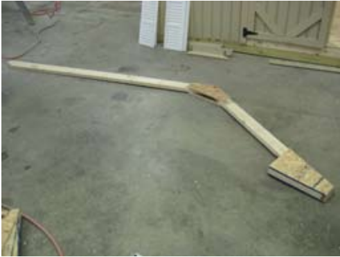
Rafter is completed and ready for installation.
