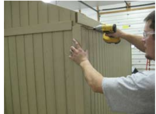
Secure trim with 1 1/4" zinc screws.
