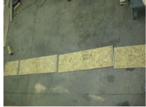
Next locate the LP siding strips as shown.
