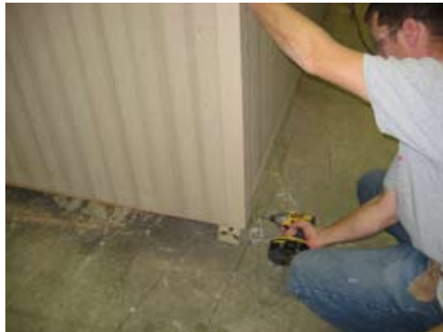
Securing trim with 1 1/4" zinc screw.
