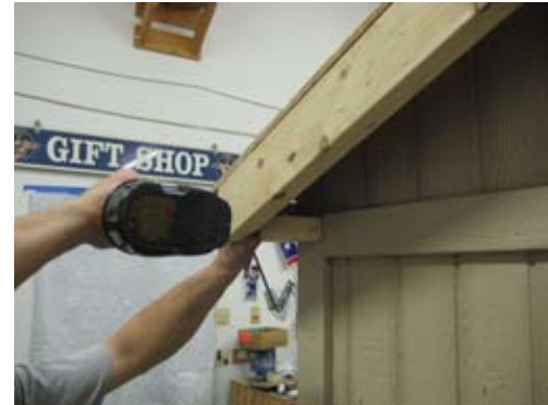
Once rake is in place secure with 2 1/2" zinc screw into rake block.
