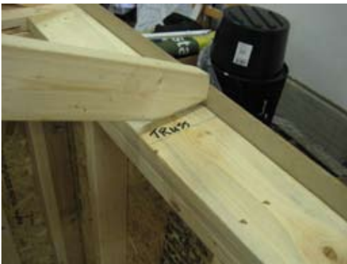
Back wall view. Plate is marked for truss location.
