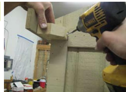
secure rake block with 2 1/2" zinc screw.
