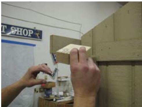
Install rake block
