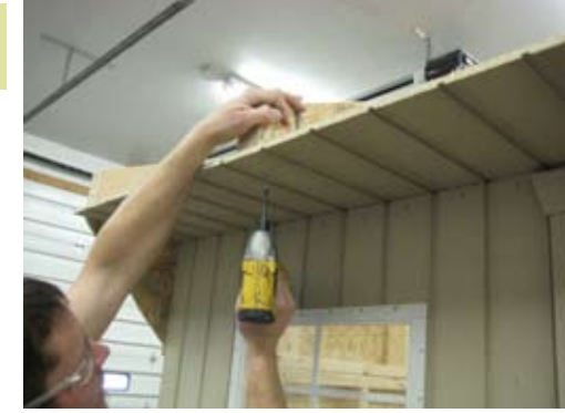
Secure with 2 1/2" screw from underneath overhang. First make sure rafter is in place.
