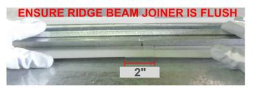
STAGE 3: TURN RIDGE CAP OVER AND MEASURE 9 27/32" FROM THE END OF EACH RIDGE CAP. PLACE TEK SCREWS IN 2" INCREMENTS FROM SAID END. REPEAT THIS PROCESS FOR THE OPPOSING HALF OF RIDGE BEAM
