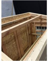
Pictured is the fastened roof purlin.
