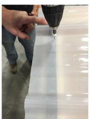
Attach using 1" white screws where holes are drilled in the roof.
