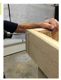
Fasten the outside of the walls together using screws.
