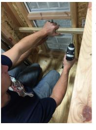
Fasten using 2 1/2" screws. And do the same to the opposite side.
