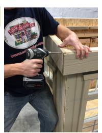
Fasten the sidewall to the back wall using 2 1/2" screws.
