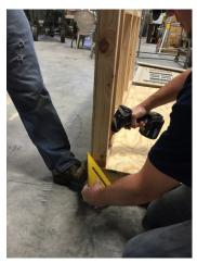
Make sure the back wall is square to the floor and fasten using 2 1/2" screws.
