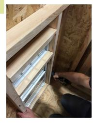
Fasten the sidewall to the floor using 2 1/2" screws. And do the same to the second sidewall.
