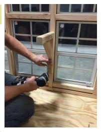
Fasten using 2 1/2" screws. And do the same for the second side center support beam. 20
