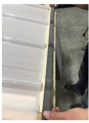
Before fastening the roof sheeting, attach the foam sealer onto the roof corresponding to the ridges in the roof sheeting.
