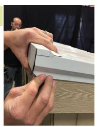
Be sure that the drip edge pieces align completely before fastening.
