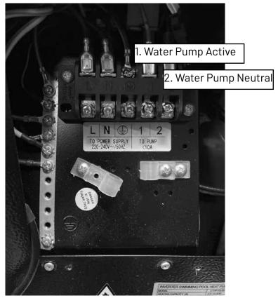
Figure 11: Electrical Connections for Single Phase Units
