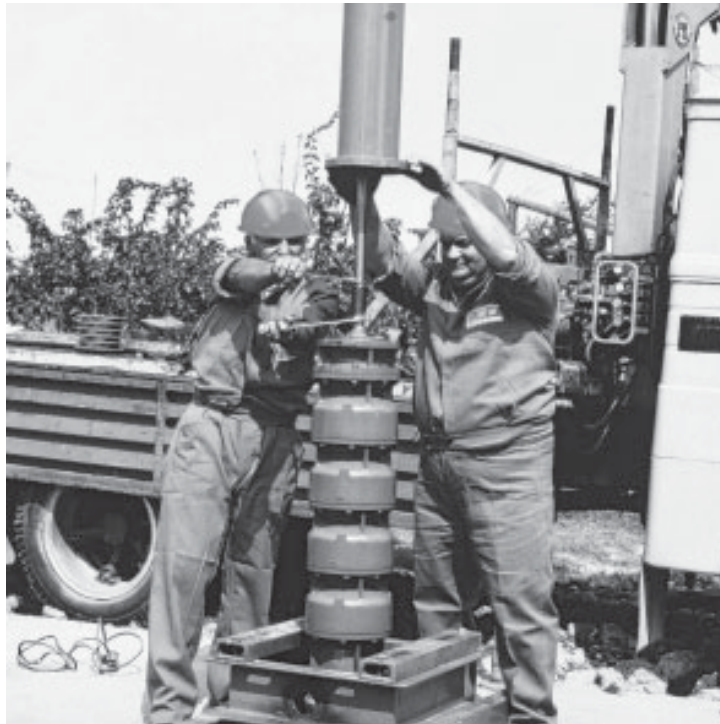
fig. 6 - Fully torque with wrenches
