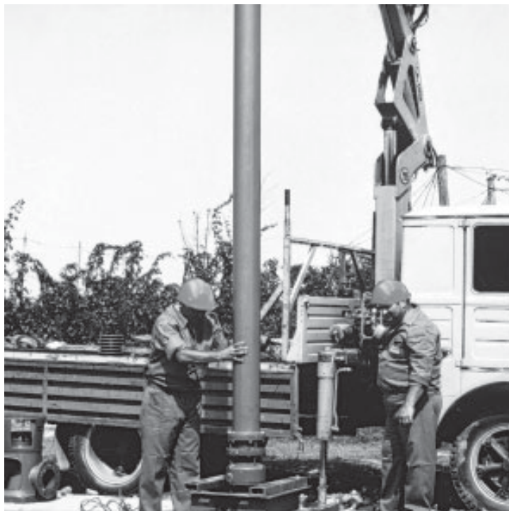
fig. 7 - Lower the assembly so that the brackets rest on the bearing frame
