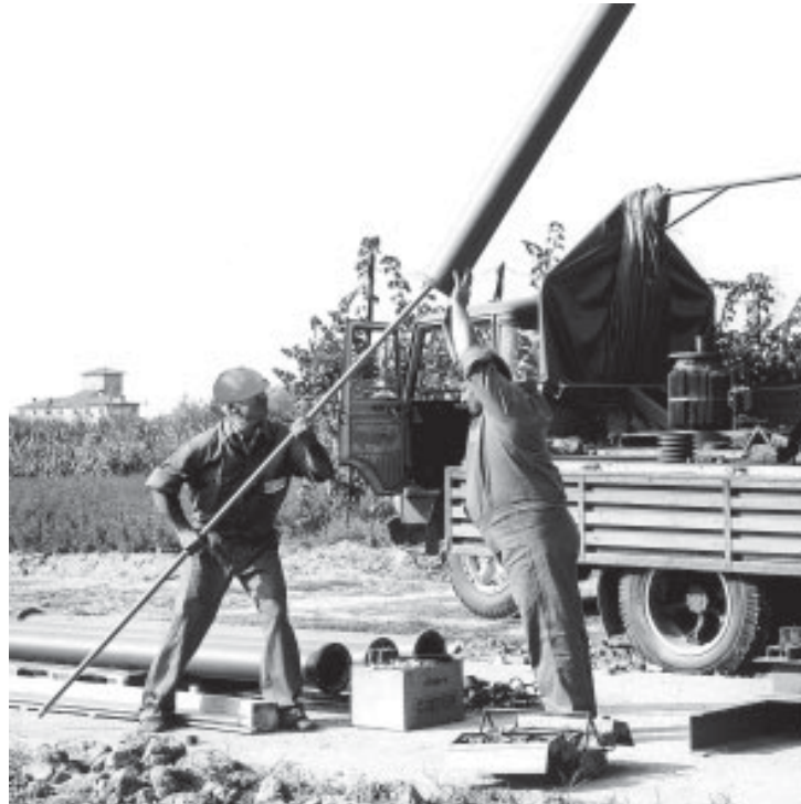
fig. 4 - Slant the pipe so as to insert the driving shaft section
