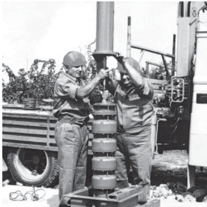
fig. 5 - Fully tighten by hand to prevent the thread from being damaged
