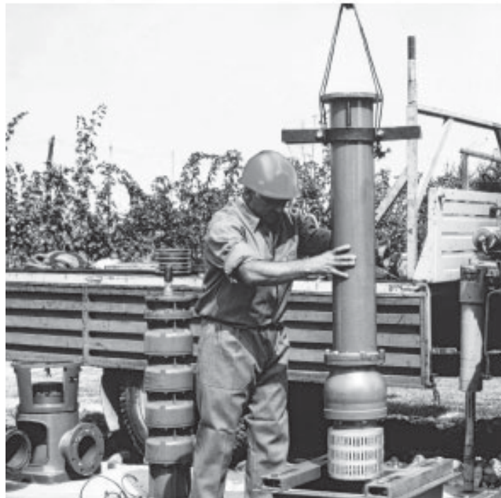
fig. 2 - Lowering the foot valve and suction pipe into the well
