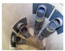
DN/OD 160 up to 400 for concrete chambers DN 1000, 1200 and 1500
