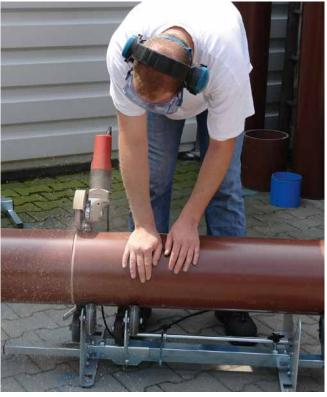
Cutting to length and simultaneous chamfering of the pipe
