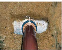
approved construction materials in rounded or crushed form as graded mixture 0 – 32 mm up to 10 cm above the crown of the pipe; Excerpts from EN 1610:2015-12 clauses 5.3.3.2 (and following) Granular Materials
