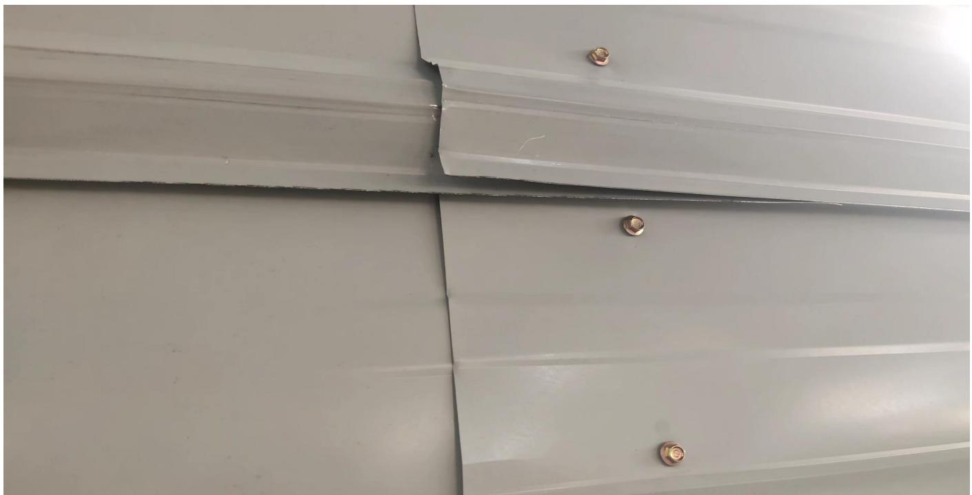
The extra part of the model A screw is used for the situation shown in the circle above, and the customer decides whether to install it, if installed, as shown in the circle below.
