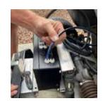
Run Tubing under cart and connect Tubing to the Mist Controller
