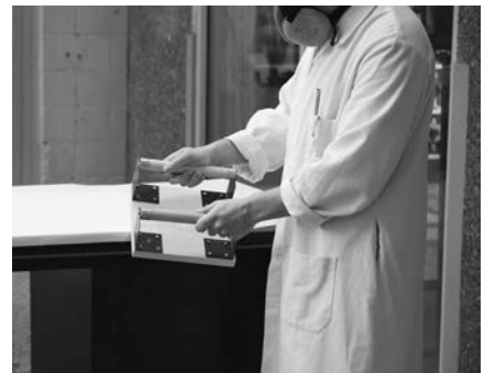
Figure 9: sanding the shelf using a large sanding block.
