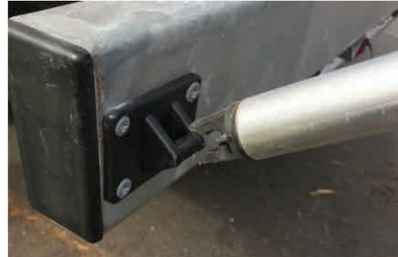
Pole 4b and bird beak plate mounting
