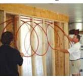
PEX tubing is looped through holes drilled in wall studs.
