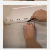
Now that the wall mural is up, it is time to **trim the edges.** Using a squeegee and a sharp scalpel, run the blade along the corners.
