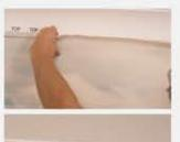
Now take the second strip and repeat the process of peeling back the the first 40-80cm of backing paper. Put the second strip up in the same way as the first. Ensure that the design is well matched up. Sometimes it is easier to work from the left edge, which touches the first strip. Don't worry if the design is very slightly misaligned as it will be very hard to spot when the mural is all up.
