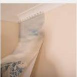
Now you can proceed to stick the rest of the strip to the wall. First you have to **remove the backing paper** by gently and evenly pulling it downwards. Be careful not to pull to hard or you might pull the top of the mural off the wall.
