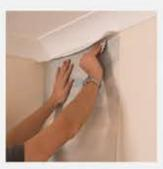
If the wallpaper sticks to itself don't worry, even if it appears heavily crinkled it can be saved by simply pulling at the edges gently to unstick it. Any crinkles will go when it is stuck onto the wall. Use a squeegee to ensure the top of the first strip is thoroughly stuck to the wall. Use the squeegee to stick the top of the mural into place.
