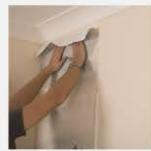
Use your hands to smooth the top of the wallpaper onto the wall. Don't worry if it isn't straight first time, you can just peel it off and try again. Use a spirit level to check that the first strip is vertical before sticking the whole strip up.
