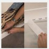
Peel off the excess mural which you have just trimmed. Use a squeegee to ensure all of the edges are thoroughly stuck to the wall. Your wall mural is now installed!
