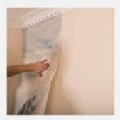
Now that the backing paper has been removed, you can press the rest of the strip onto the wall. Starting at the top, smooth your hand down the centre of the strip all the way to the bottom. Working from the middle outwards press the rest of the strip firmly onto the wall.
