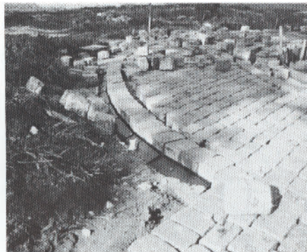
PAVE EDGE INDUSTRIAL takes a little more work to make curves.
