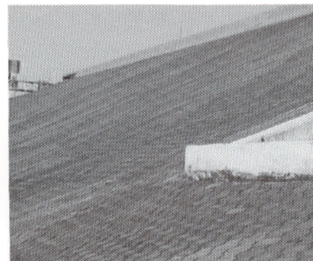
Photo #4: Who said Pavers could not be set on a steep grade?
