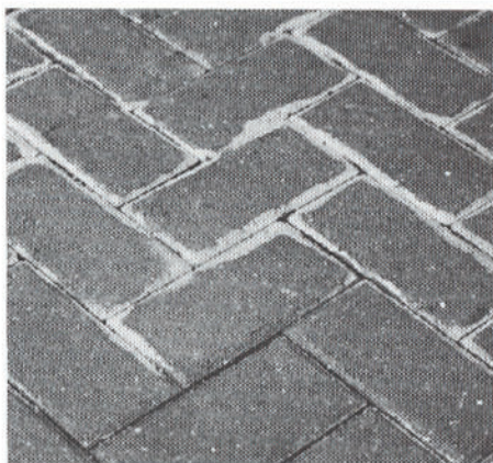
Tech Tip #1: "Sealer Glazing" can rear its ugly head if you're not careful.
