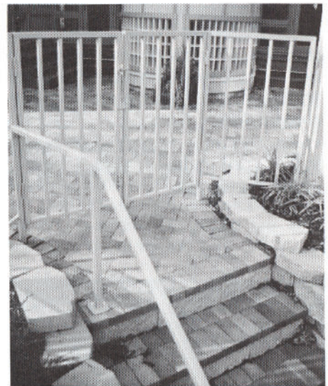
LEXEL adhesive was used on the steps.
