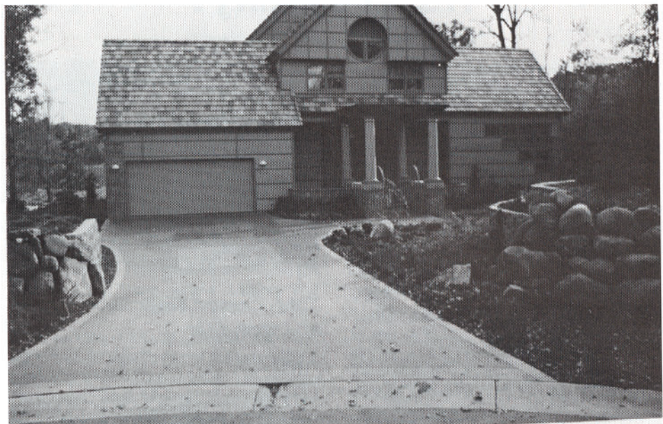
Completed — "Home of the Future" Brick paving
