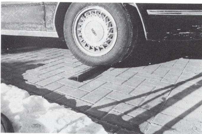
PAVE EDGE stands up to direct load of full size car.
