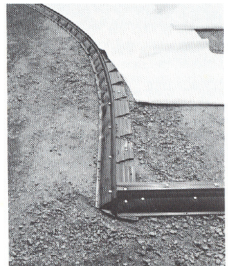
PAVE EDGE INDUSTRIAL can be relief cut to go around radius, however, it will require a substantially longer time.
