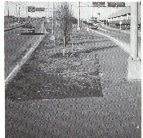
The project consisted of new walkways and pavement edges in areas around the main terminal building.
